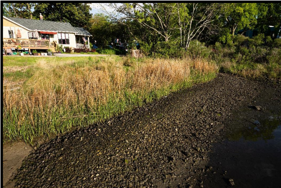
Knitting Mill Creek resident Tara Honey worked with Elizabeth River Project to convert her eroding shore into this “living shoreline.” A connected corridor of such habitats is well-underway.
