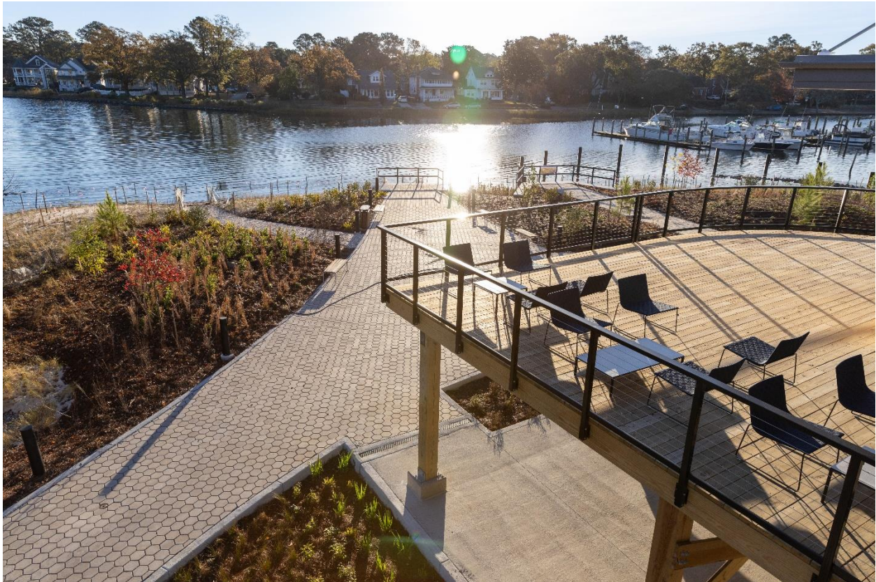
Elizabeth River Project’s Ryan Resilience Lab, overlooking Knitting Mill Creek, demonstrates stewardship of the creek and the Elizabeth River.
